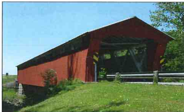
McColly Covered Bridge 13-1.56 over the Great Miami River
