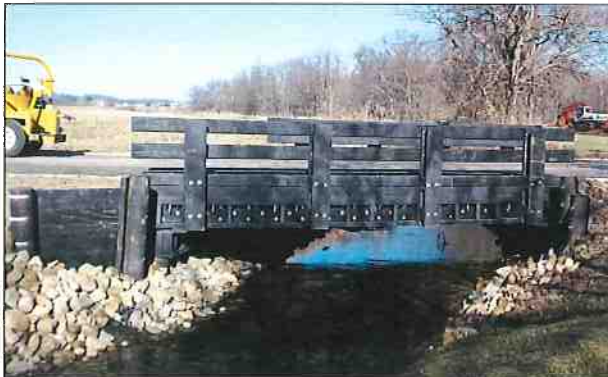
Bridge 174-0.56 over the Onion Ditch
